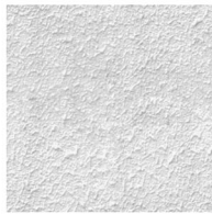
2. ORIGINAL PEBBLE AND DASH RENDER TO BE RETAINED AND RESTORED WITH SELECTED LIGHT GREY PAINT FINISH
